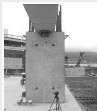
激光仪校准梁之XY向
